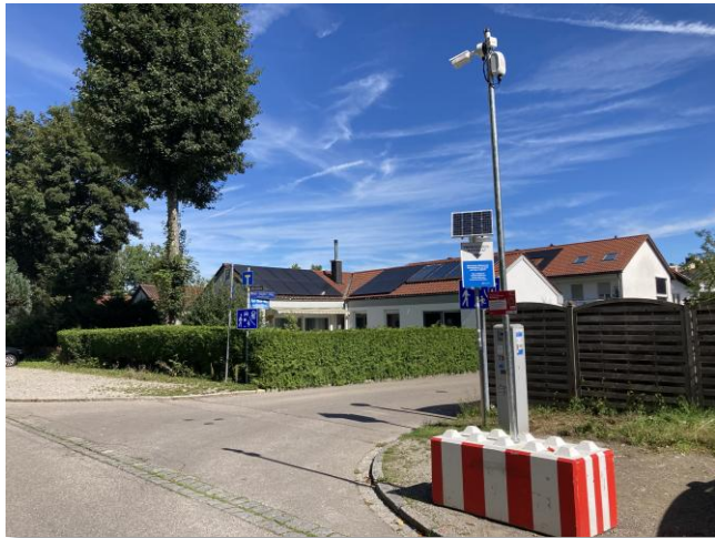
Foto: Smart City, Parkraummonitoring am Illerdamm
